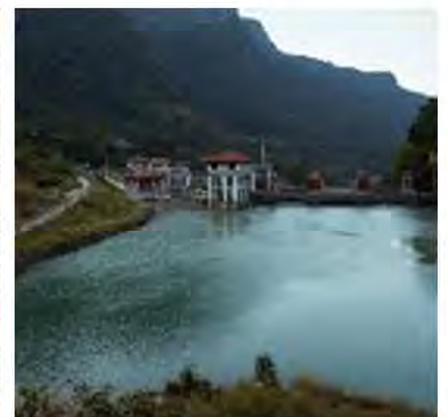
Figure 2 Upper Marsyangdi A hydropower Plant with Reservoir in Lamjung.
